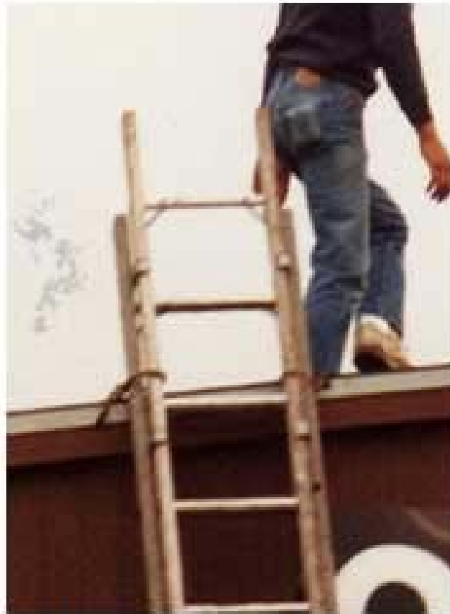
Ladder secured to roof.
