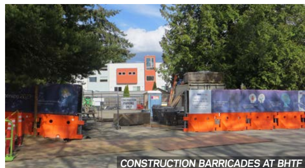
CONSTRUCTION BARRICADES AT BHTF
