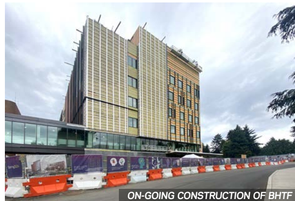
ON-GOING CONSTRUCTION OF BHTF
