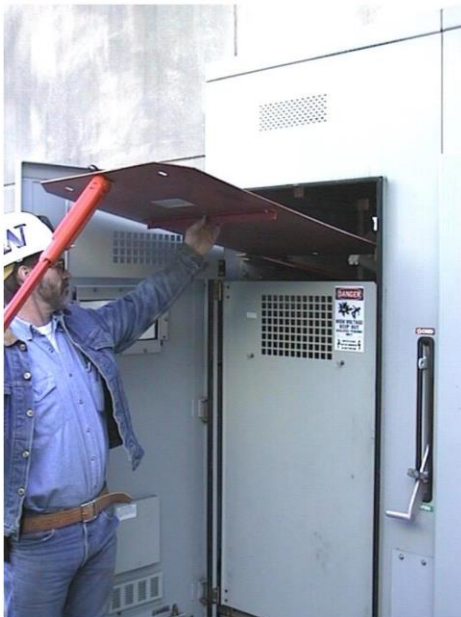
16K – Figure 3 Isolation Barrier Being Inserted
