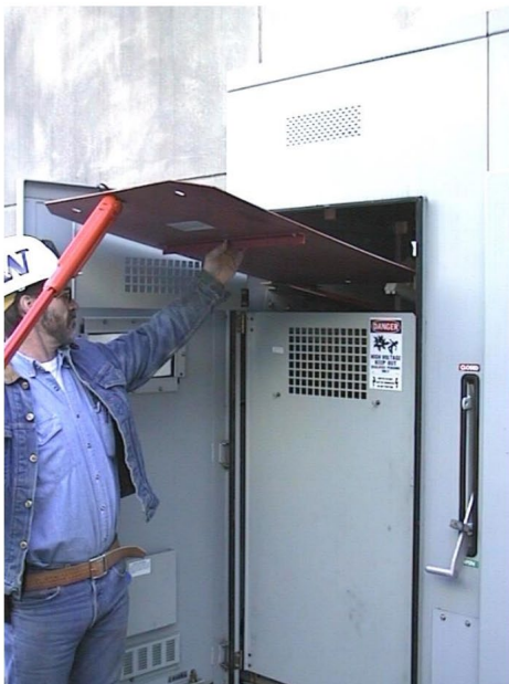
16K – Figure 3 Isolation Barrier Being Inserted
