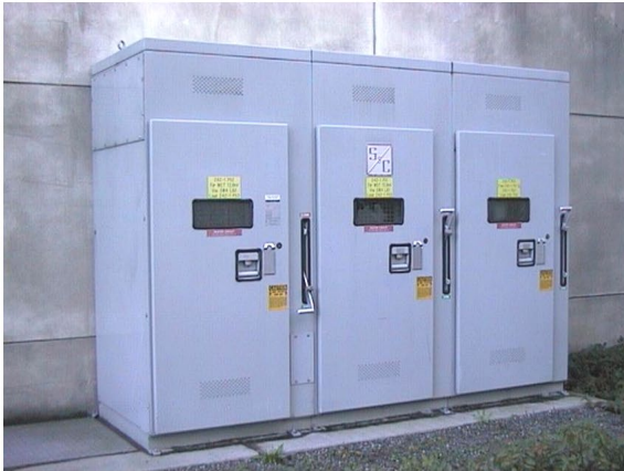
16K – Figure 1 Primary Select 3-Bay Switching
