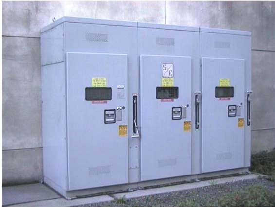
16K – Figure 1 Primary Select 3-Bay Switching
