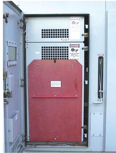
16K – Figure 2 Isolation Barrier in Storage Position
