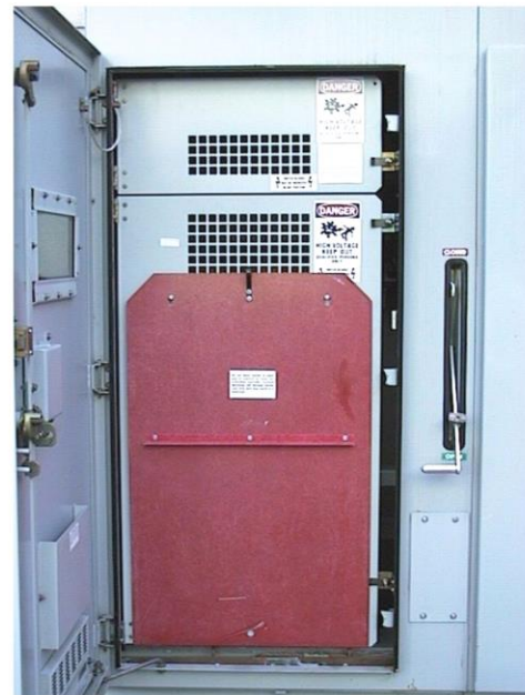
16K – Figure 2 Isolation Barrier in Storage Position
