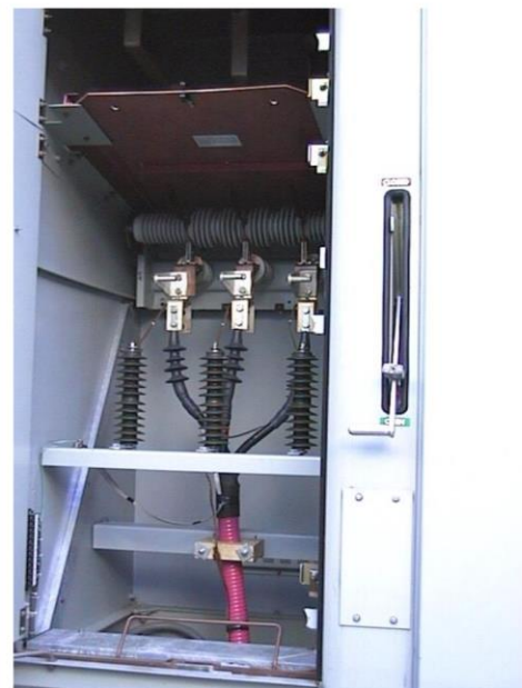
16K – Figure 4 Barrier Isolating Switch
