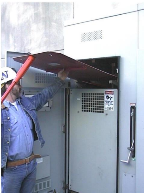
16K – Figure 3 Isolation Barrier Being Inserted
