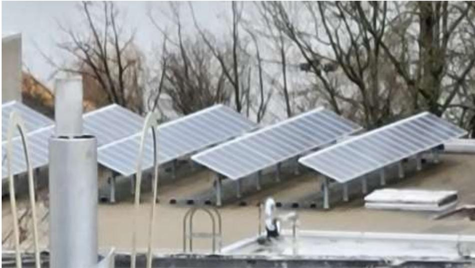
2. Photovoltaic panel arrays shall be grouped into racks or frames to minimize roof penetrations.
