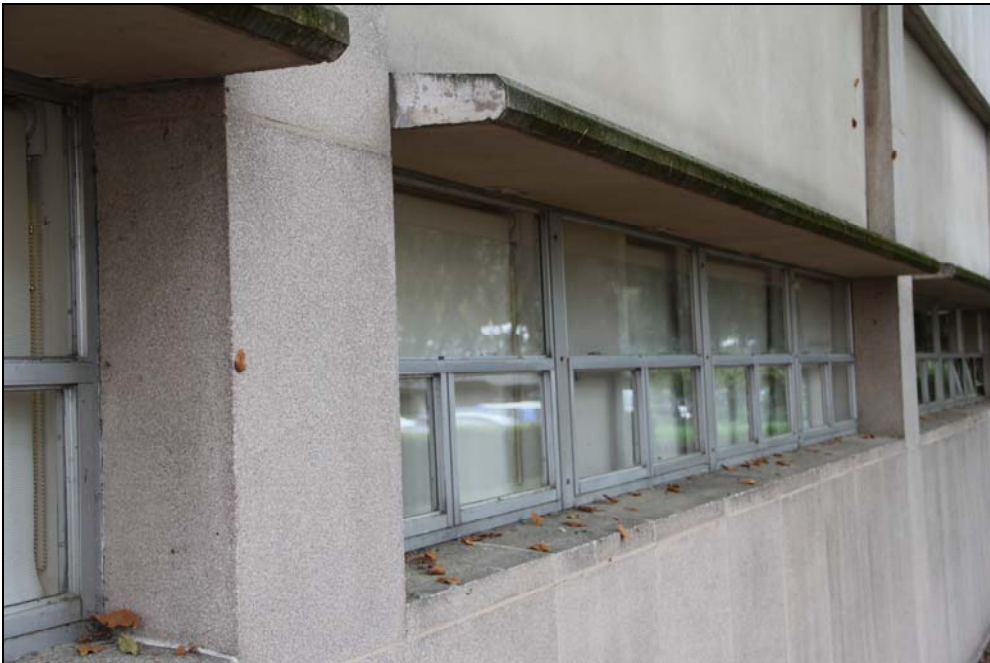
Figure 17. Below, detail view of the windows and concrete canopy on the north facade. The original design featured glass block as a glazed infill above the building's deeply inset aluminum frame windows.
