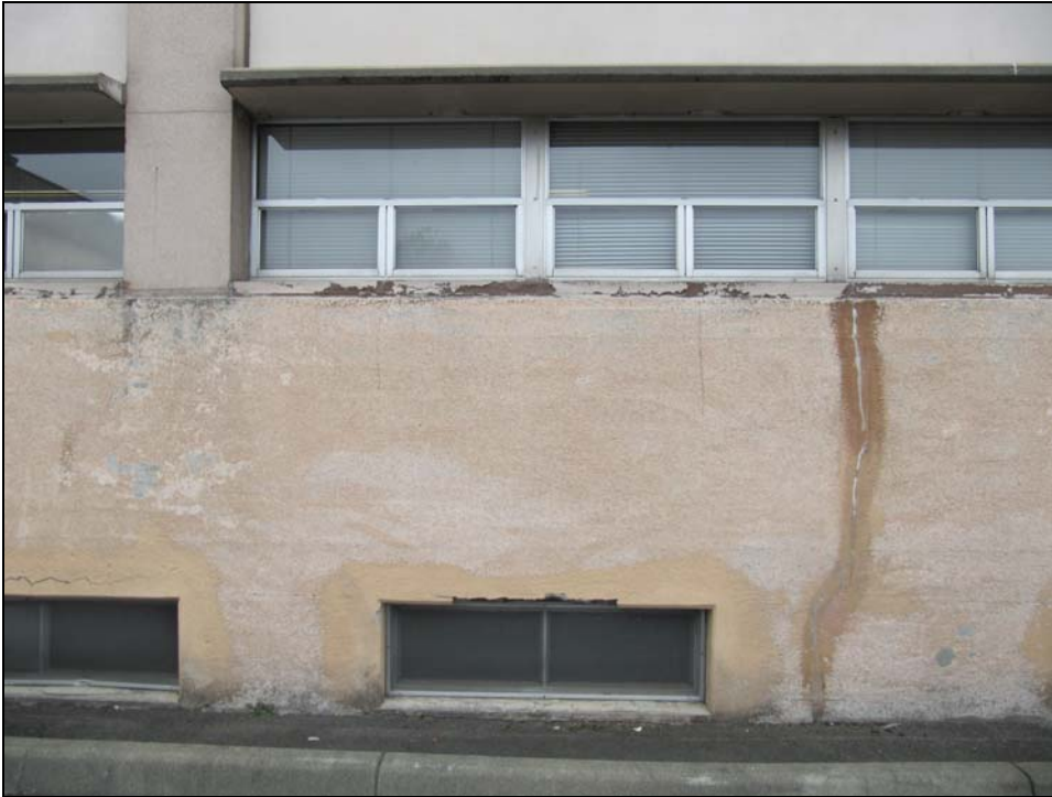
Figures 18. & 19. Above and left, detail views of current conditions on the south side of the former Fisheries Center. This face of the building is exposed to wind-driven rain and sunlight.
