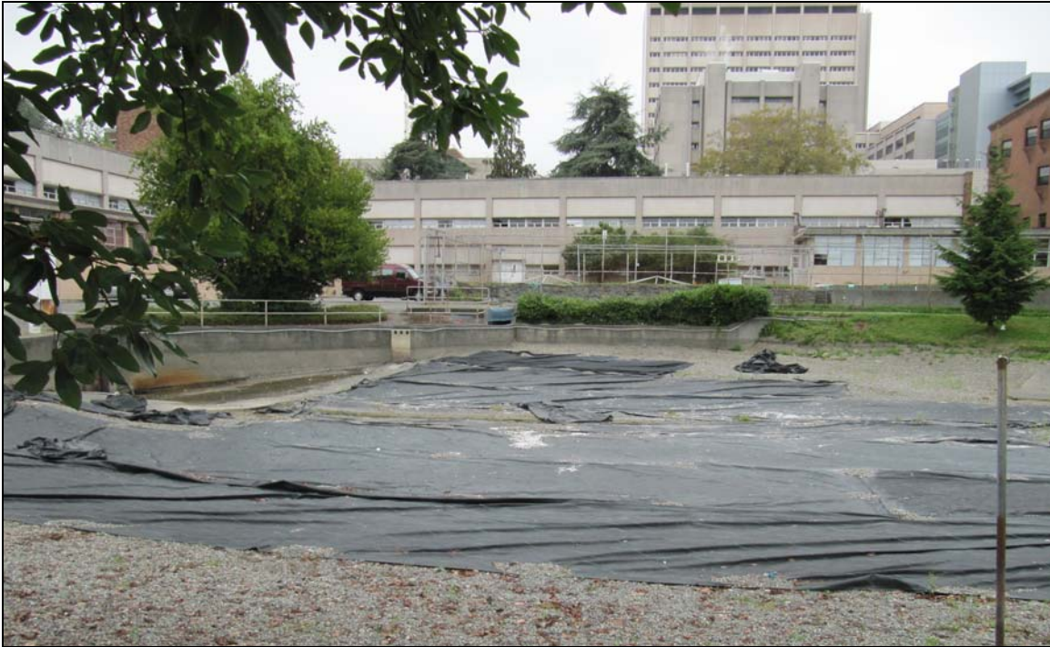
Figure 12. Above, view looking north at the south facade and main wing of the former Fisheries Center and the fish pond from the edge of Portage Bay. Parts of the UW Medical Center are visible in the background.
