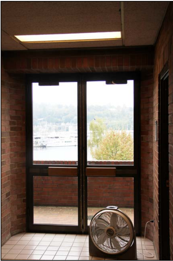
Figure 32. Above left, view looking south at the existing anodized aluminum frame access door and small balcony at the south end of the top floor. Occupants open the door and use a small fan to help ventilate the interior.
