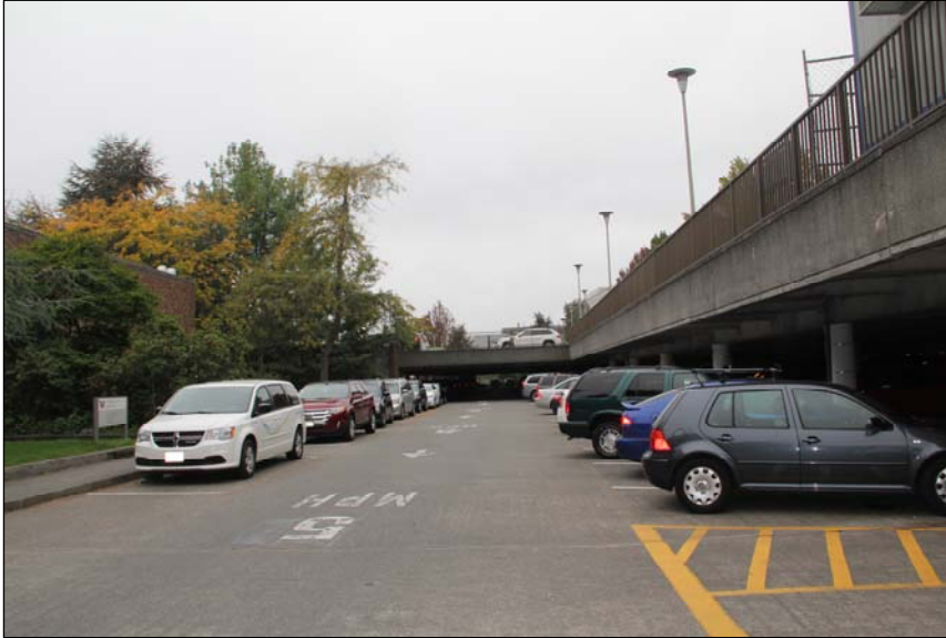
Figure 10. Above, view looking west in front of the building at the nearby parking lot and garage structure.
