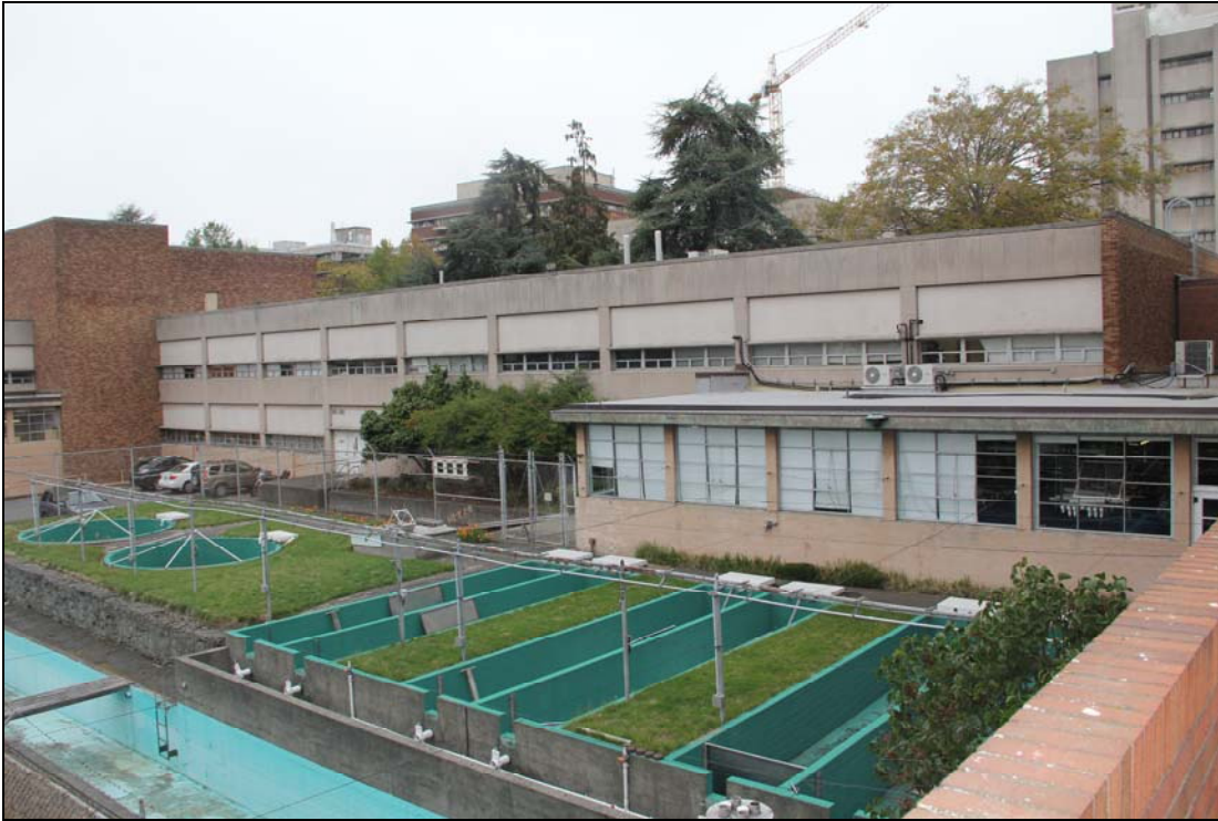
Figure 14. Above, view looking northwest at the fish pond, single-story hatchery section and portions of the south and east facades of the former Fisheries Center.
