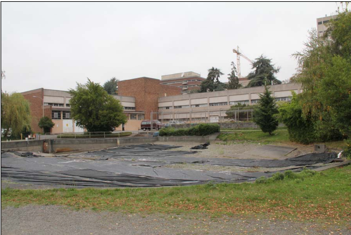
Figure 13. Below, view looking northeast at the south and east facades of the main and west wings.
