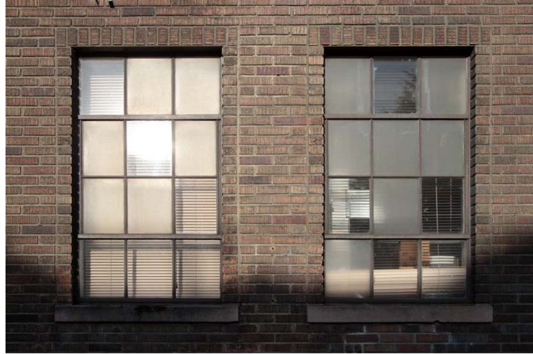
Original Windows – East Side
