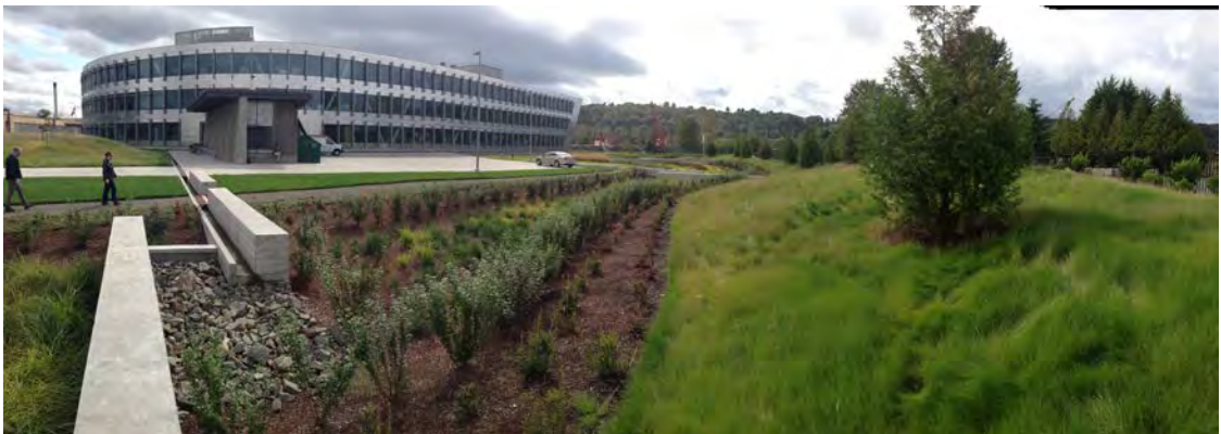
Example Large Bioretention Facility,, Seattle, WA
