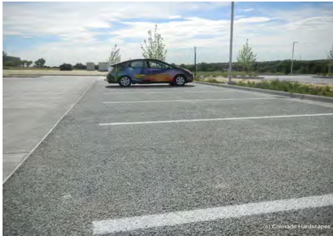
Example Porous Concrete
