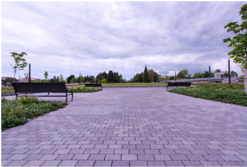
Porous Paver System Example, Montlake Triangle
