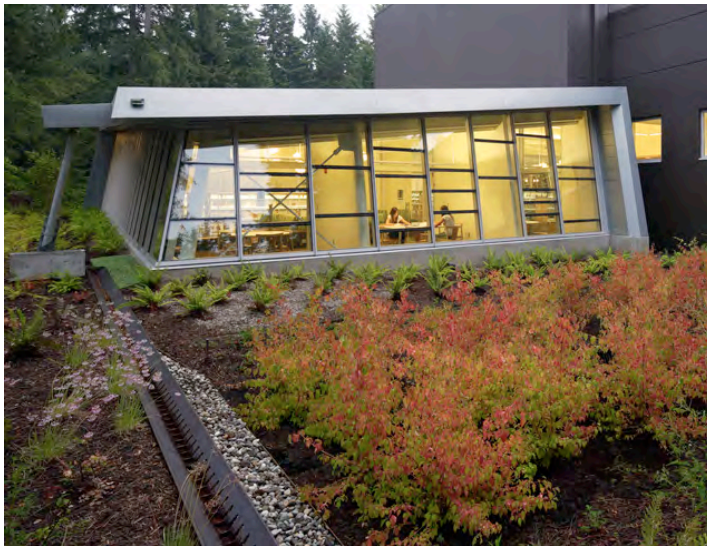
Non-Infiltrating Bioretention, Federal Way Library
