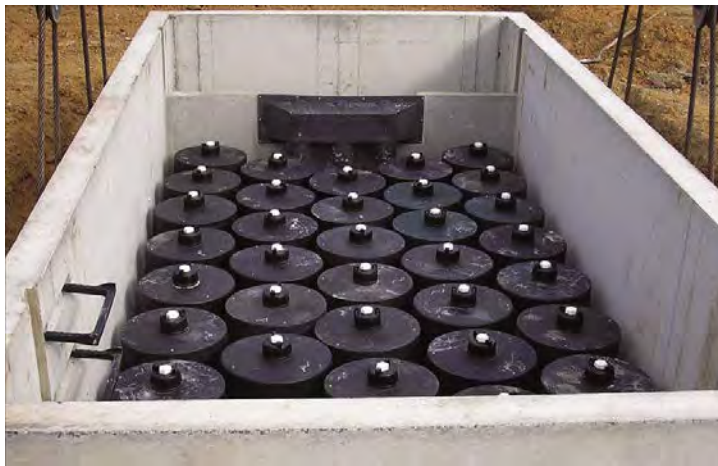
Example of Proprietary Filter Media Cartridge System
