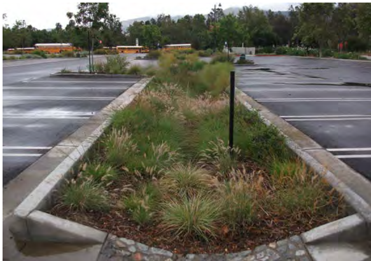
Example of Parking Lot Biofiltration Swale with Tall Grasses
