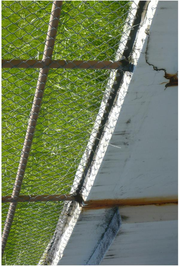
Damage Caused by Guardrail Mounting
