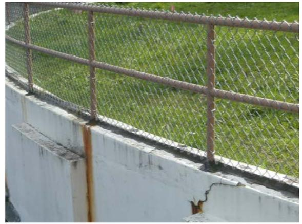
Damage Caused by Railing Mounting
