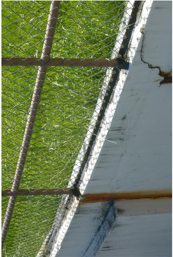
Damage Caused by Guardrail Mounting
