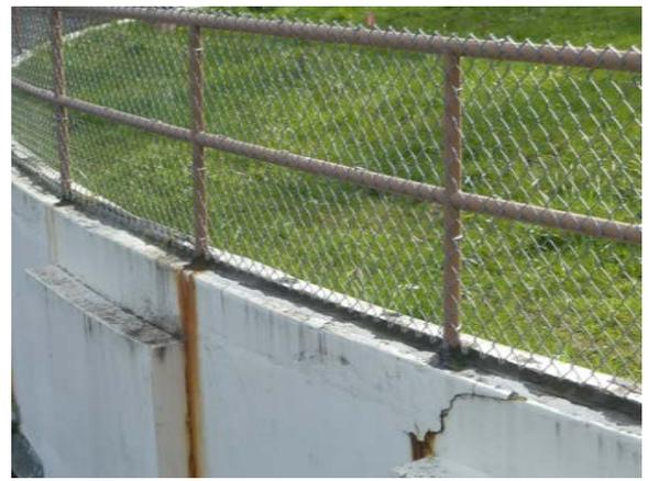
Damage Caused by Railing Mounting
