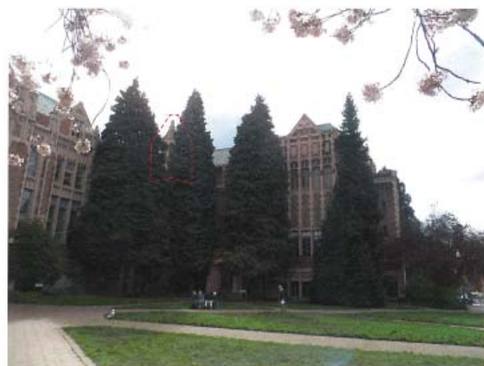
Gowen Hall - DRB review concluded a tree removal would benefit both access for tower repairs and restore the view of the building from the Quad.
