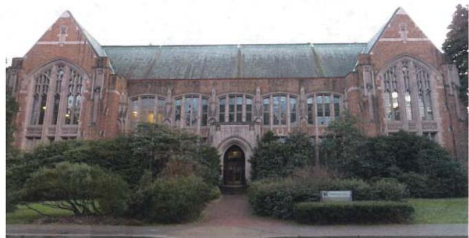
Photograph of Existing North Elevation
