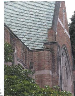
Photograph of Existing Copper Saddle Flashing visible from Stevens Way
