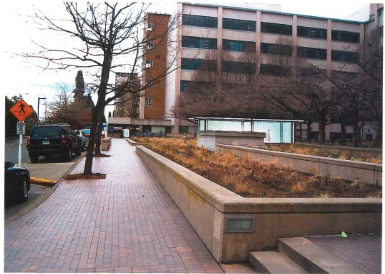
View of stair canopy from West
