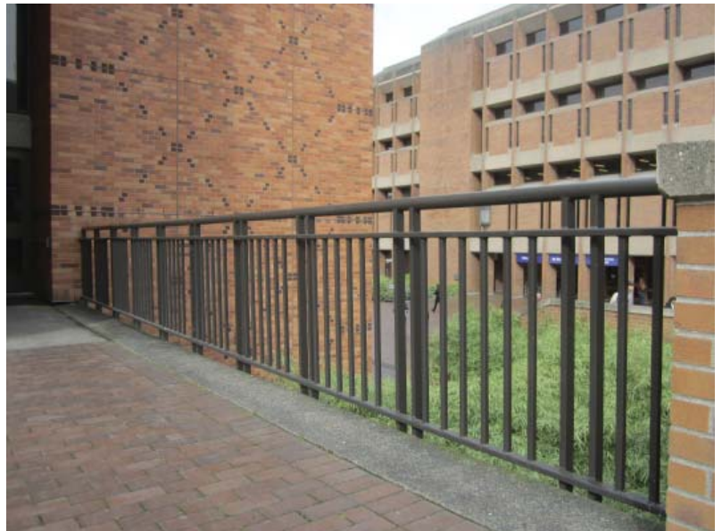
Meany Hall Guardrail - The new handrail picks up the dark brick accent color in Meany Hall and continues the use of a dark bronze common University color for metal work.
