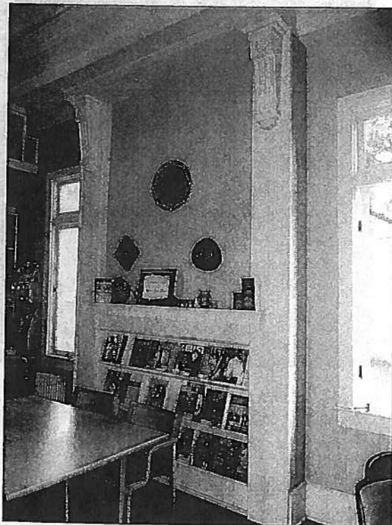
Left: Casework located in place of the original fireplace at the interior west wall in the Women's Center Library.
