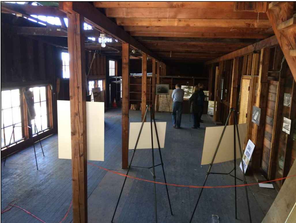
Figure 26. Interior view looking west in the mezzanine at the north end of the building.
