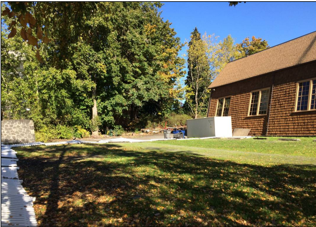
Figure 12. Looking northeast across the west side yard. Mature trees and a lower grade separate the building from the large E12 parking lot farther north.
