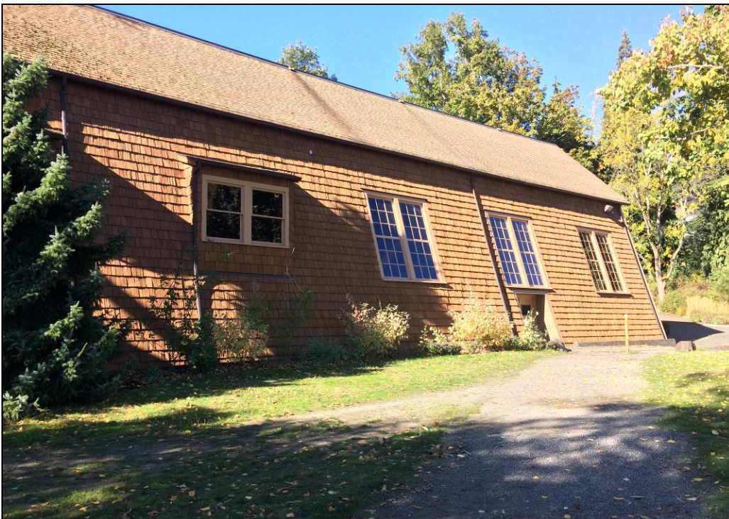
Figure 16. Looking northwest along part of the east façade and side yard.
