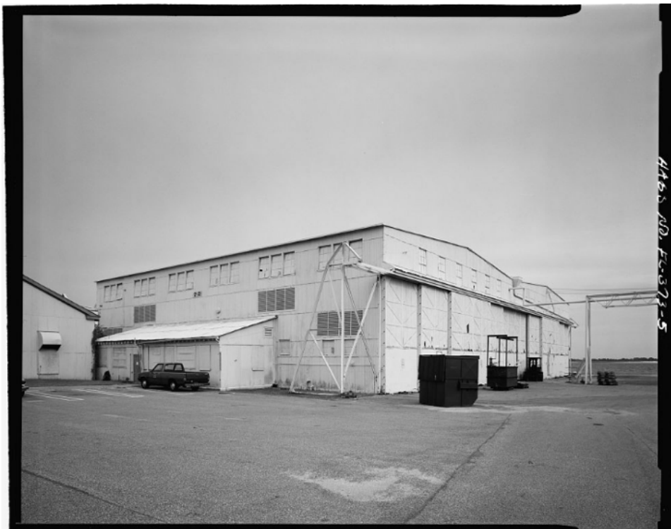
Figure 32. Building 72 was a double-gabled seaplane hangar built in 1916-18 at Pensacola Naval Air Station. The building has been demolished, but was documented to record its history and significance as part of the Historic American Buildings Survey (HABS).
