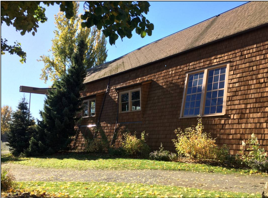
Figure 15. Looking southwest along part of the east façade and side yard.
