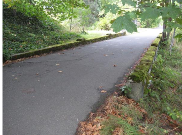
Looking NE on trail, bridge visible (top portion of original parapet) 2013
