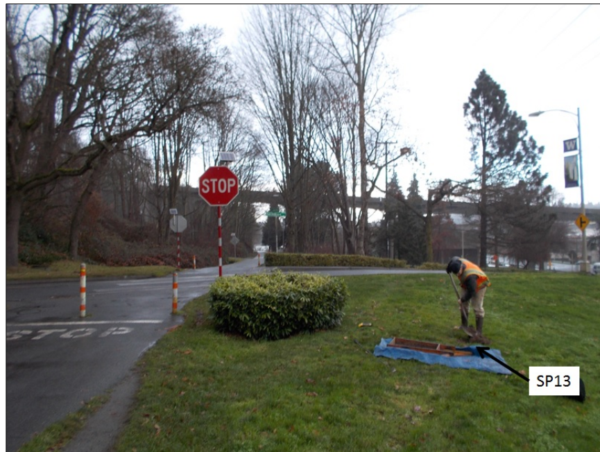
Figure 7-8. Overview of SP13 location, view north.
