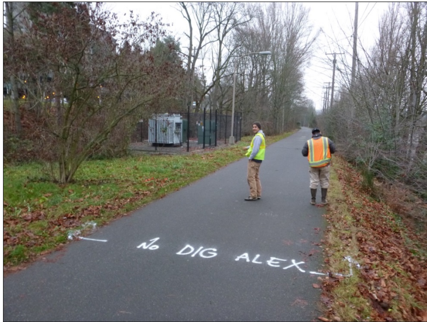
Figure 7-3. Note electrical facilities at left, view north.
