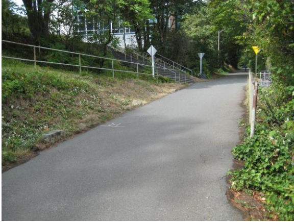
Looking north along bridge deck 2013
