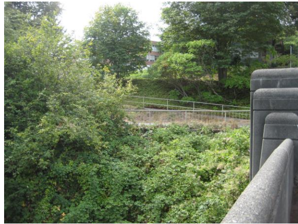
Looking west toward the bridge, view from the Pavilion/Stadium Overpass 2014
