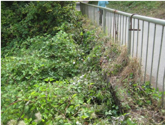
Looking SW along eastern edge of bridge 2013
