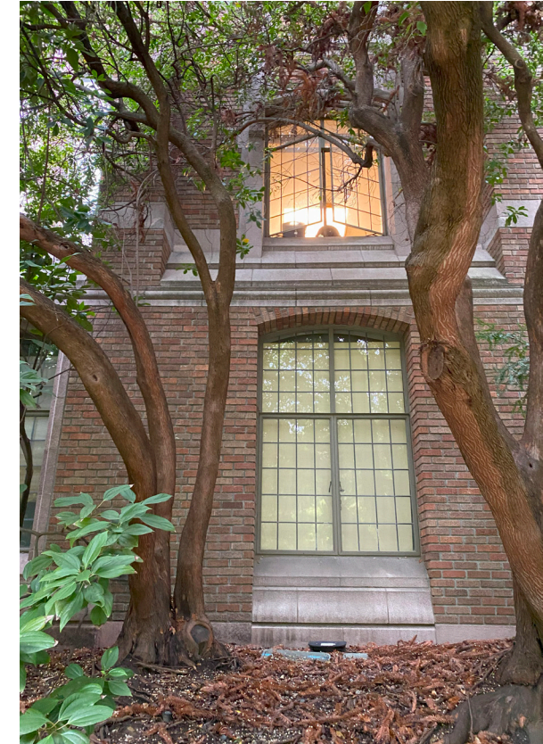
Existing condition of 1970's Infill after removal of arcade
