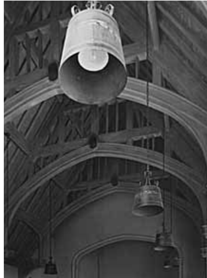
Original Light Fixture at Auditorium
